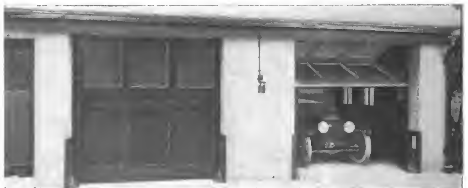
Fold-up door for garages, which is out of the way when open
